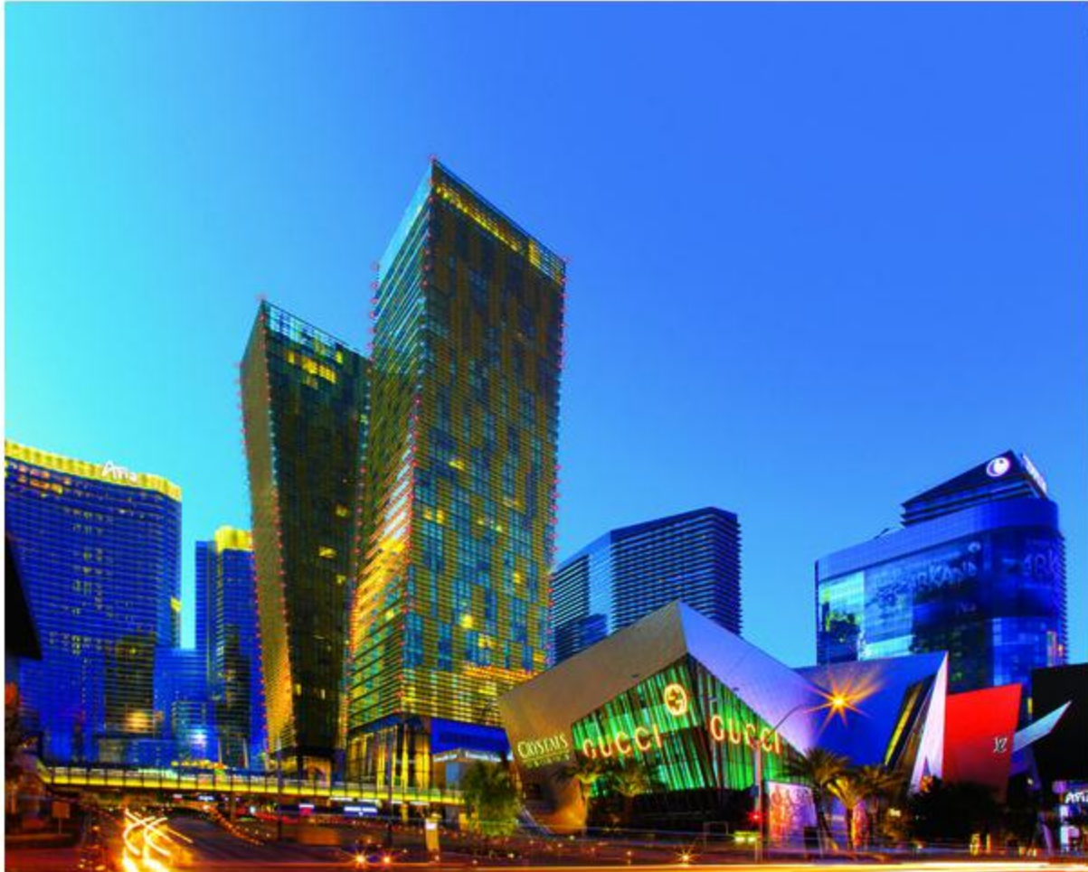
Built at opposing five-degree angles for a leaning, peek-a-boo effect, and designed by Murphy/Jahn Architects of Chicago, Veer Towers are for residents only.
